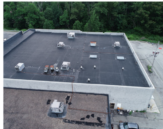
#6: VIEW FROM SOUTH SHOWING SECTIONS A,B,D
